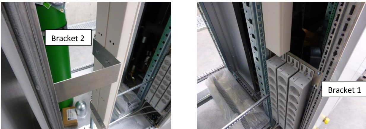
The rear view of Slave LLRF racks for L2&L3 - cables ducts for signals (left) and AC/DC cables (right).
