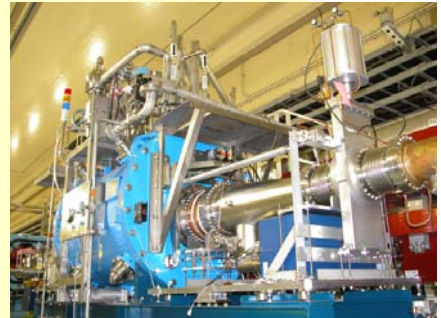
The superconducting cavities will be upgraded to absorb more higher-order mode power up to 50 kW.
