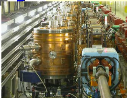
The state-of-art ARES copper cavities will be upgraded with higher energy storage ratio to support higher current.
