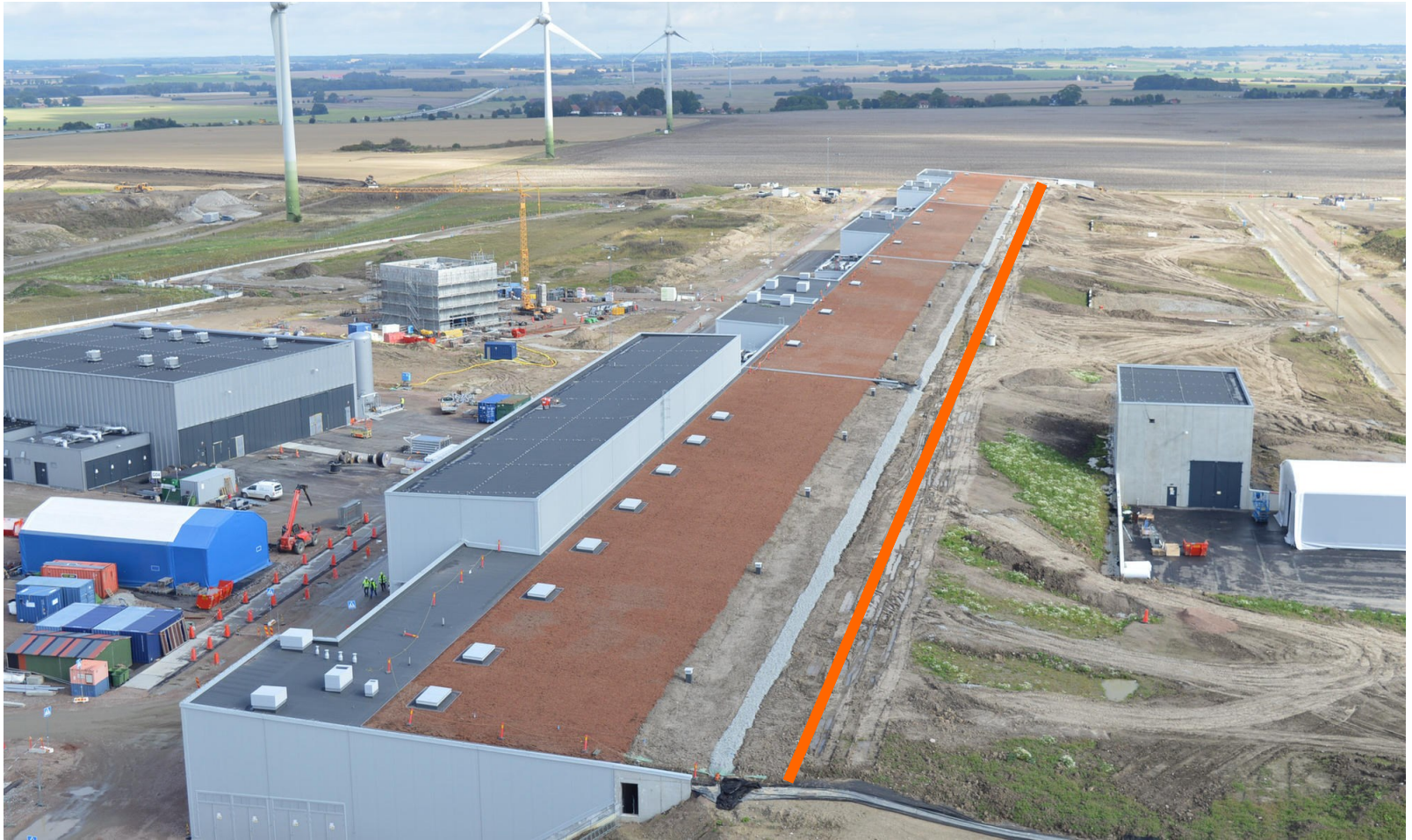
Klystron gallery and berm over tunnel.
