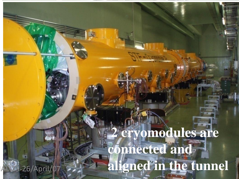
Setting the module on the tunnel floor
