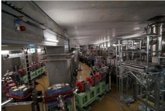
**Compact ERL (cERL)** has been constructed in 2013 at KEK to demonstrate energy recovery with low-emittance, high-current CW beams of more than 10 mA for future multi-GeV ERL & CW X-FEL.
