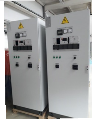
Sextupole & steerer power converters
