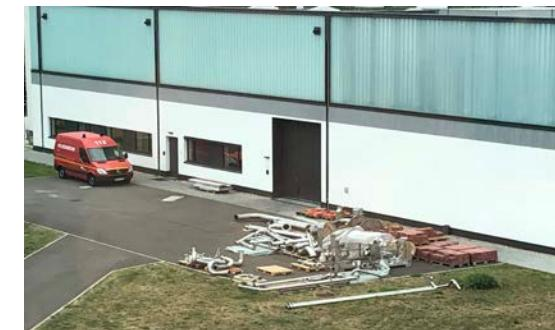
Rust in de-ionized water cooling circuits of bERLinPro, nearly complete system needs to be exchanged
