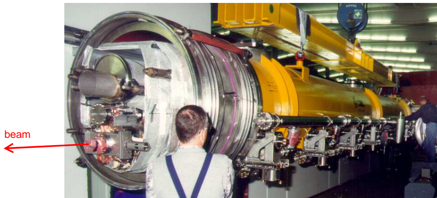
module installation in FLASH (2004)
