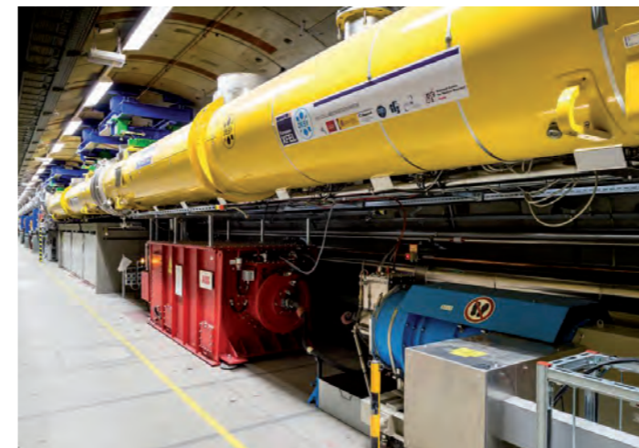
View into the tunnel of the 1.7-kilometre-long superconducting linear accelerator of the European XFEL
