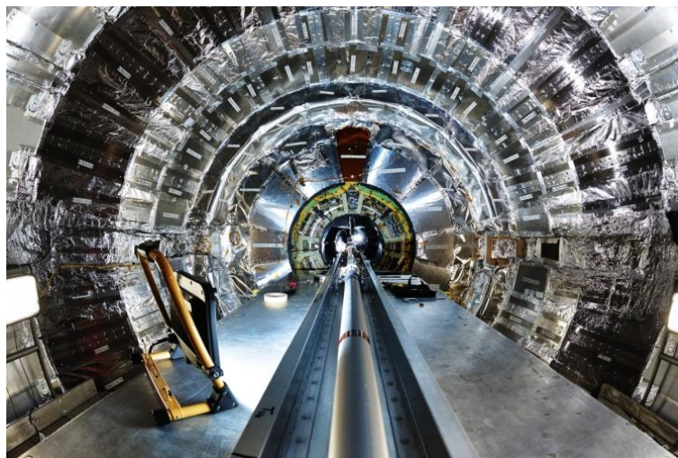
New beam pipe installed
