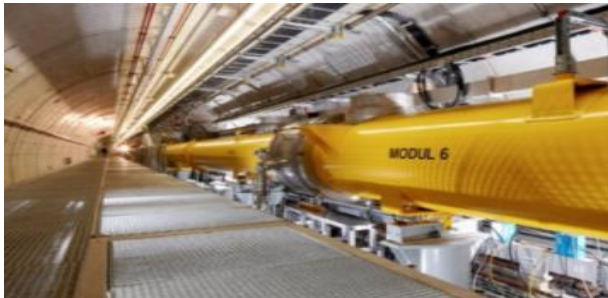
TESLA type superconducting accelerating modules 1.3 GHz
