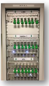
BKR interlock keys for labyrinths and media shafts (L/MS), Injector 1 and XTL
