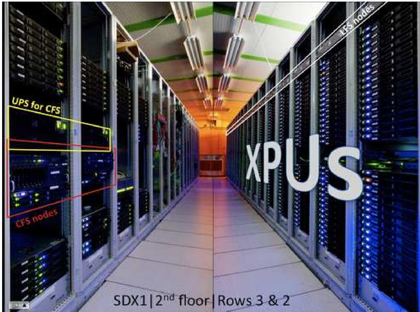
XPU S = Interchangeable processing units (can be used for L2 or EF)
