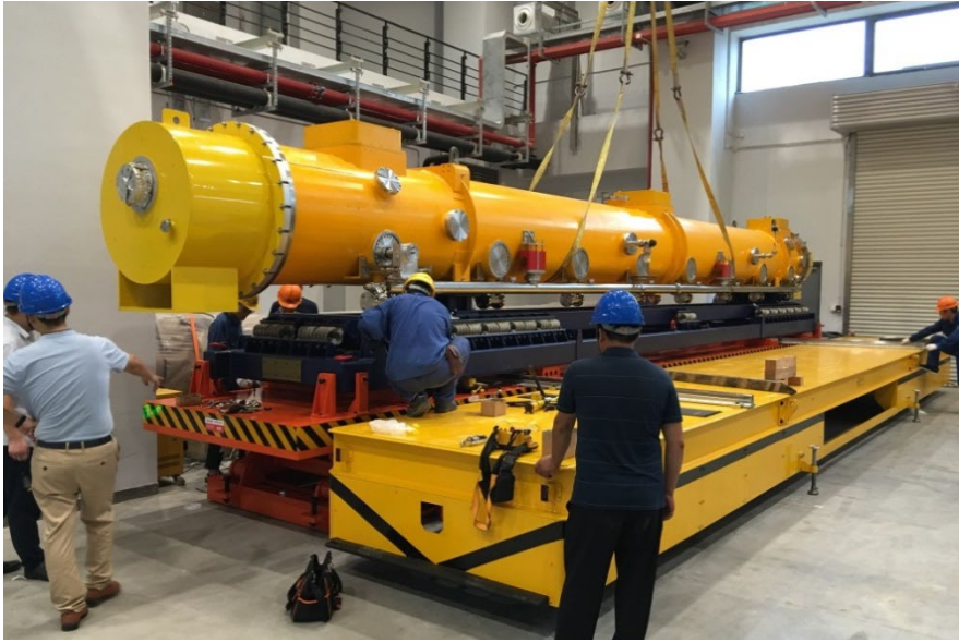
Tools for CM installation
