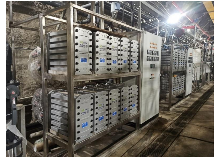
Water system almost ready for commissioning
