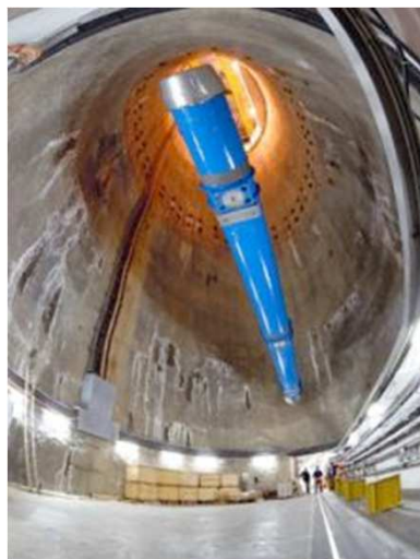
April 2008 Last dipole down (Total: 1232 dipoles)
