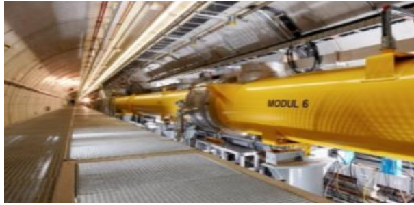
TESLA type superconducting accelerating modules 1.3 GHz
