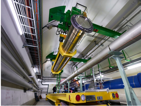
One of the two spare LHC's beam dumps is removed from the tunnel for upgrade work in preparation for Run 3 (Image: CERN)
