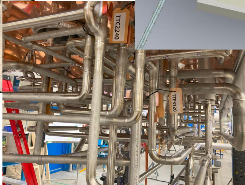
The new cryobox for He distribution.
