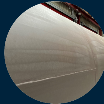
Tower first coat
