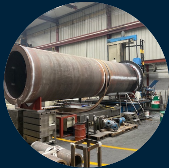
Complete welded tower
