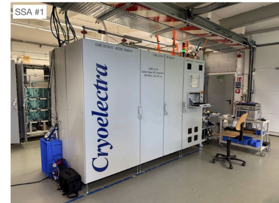
First of 7 x 120 kW solid-state amplifiers delivered to Diamond
