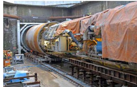
10.01.2011: TULA in der Baugrube Osdorfer Born
