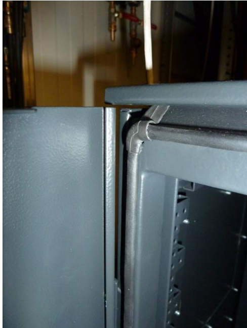
Fig. 9. Only rubber sealing, no EMI sealing (copper mesh).
