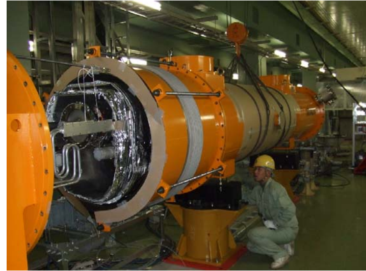
Placing the cryomodule on the stand in the tunnel.
