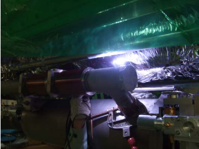
Welding the helium supply pipe by the company welder.
