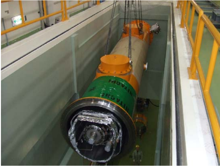
Transporting the cryomodule into the tunnel.
