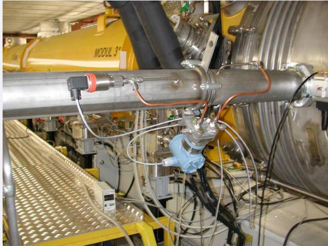
Venting system beam-pipe-vac DN 100
