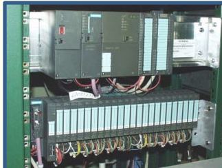
The SIMATIC S7 is the interface between the control system and the installed hardware. It also manages the interlock signals and drives the motors which allow for changes to the pulse compressor tuning.
