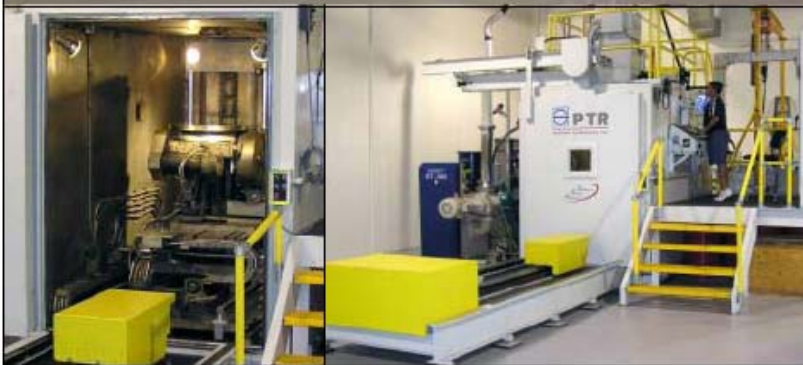
Figure 3: EB Welding System at AES
